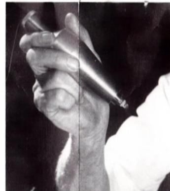
After removing barrel, (Figure 2), screw light into opening (Figure 3) until bulb is securely tightened.
