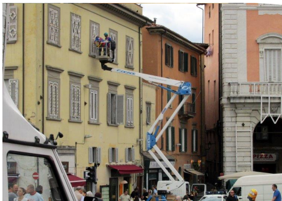
Installing the candles
